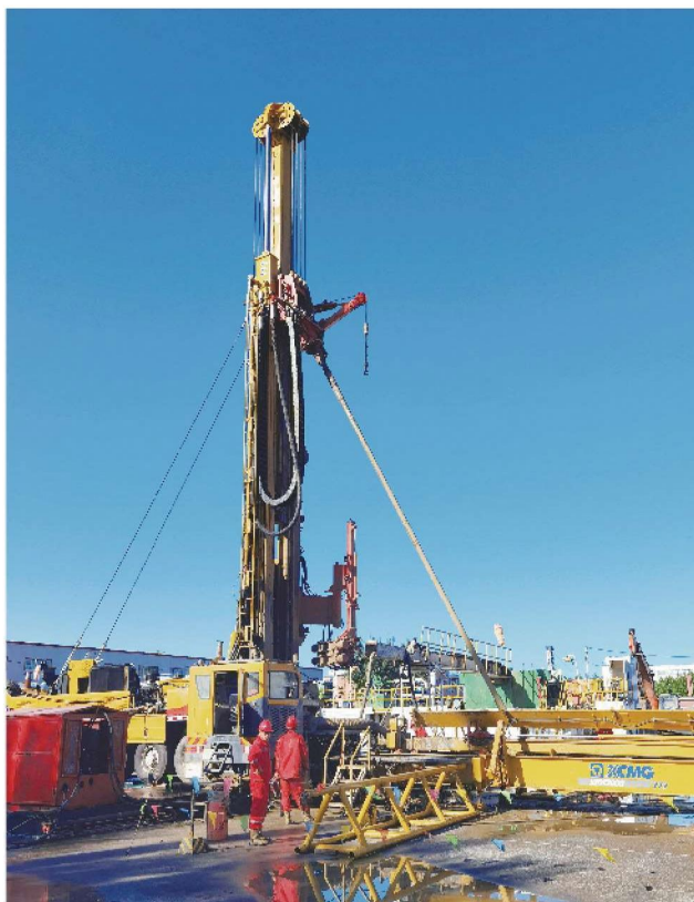
Deep well drilling rig Liaoning ultra-shallow and ultralong horizontal well construction
