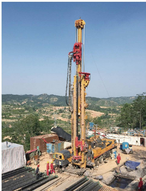
Deep well drilling rig Shanxi coalbed methane well construction
